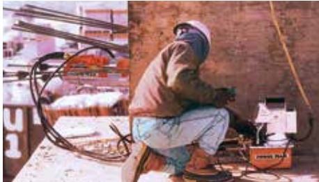
The PE60 used for pre-stressing.
