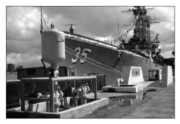
Fuel loading absorbs shock from pump startup and stopping
